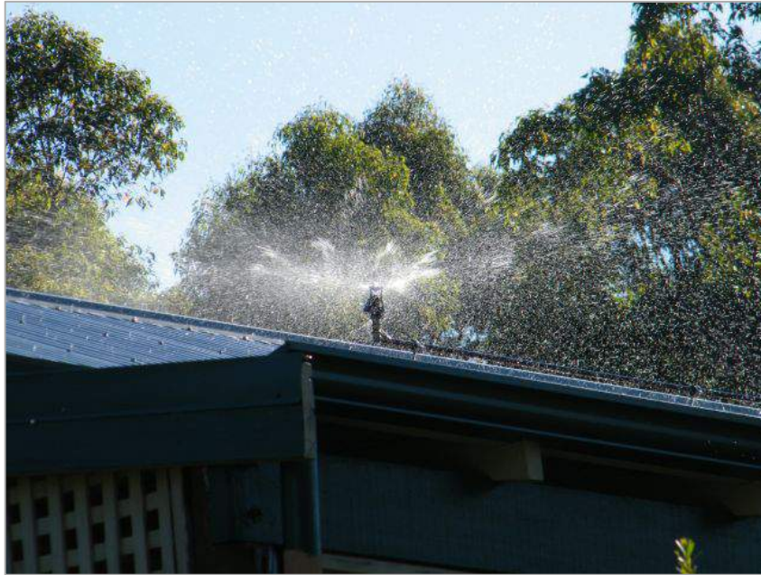
Figure 3. Example of a sprinkler used on a rooftop to protect the building from ember showers. Photo credit: Small Farm Services, Australia.
